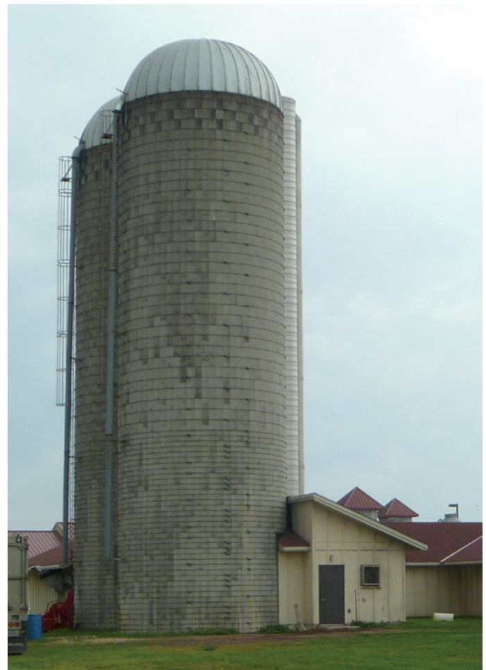
Figure 5. Concrete stave tower silos.
