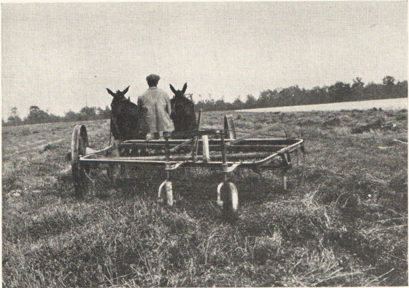
USE OF SIDE DELIVERY RAKE IN MAKING CRIMSON CLOVER HAY.
